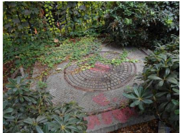
Photo #22: Transformer vault
